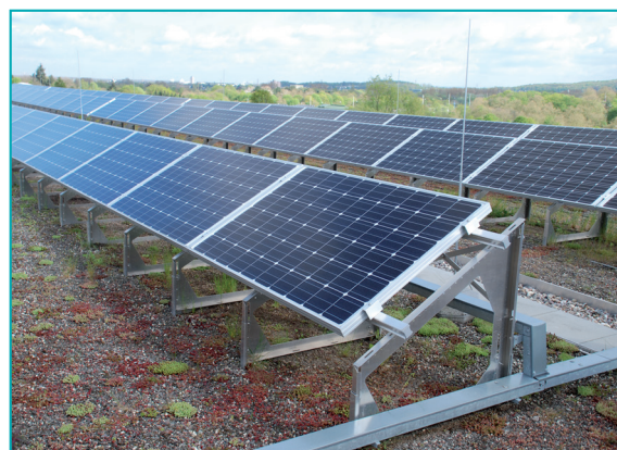
Combination of green roofs and photovoltaic panels on the roof of the Environment Ministry
